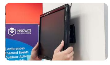
**Step 11**Once the bracket is attached to the back of the monitor, hook the TV on to the fixed bracket on the Exhibit panel.
